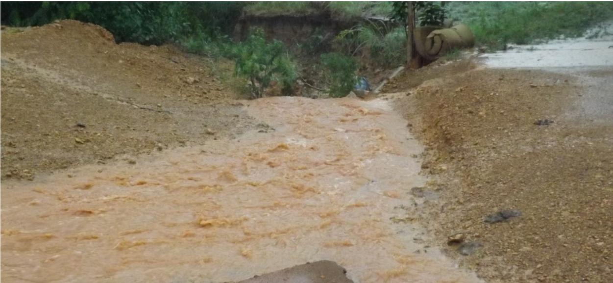
Figure 10 - Erosive feature (gully) observed during the implantation of the Jardim Nova América subdivision (Photograph: Lucas B. Souza, March/2015).
